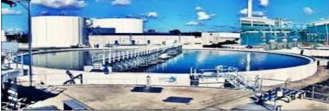
Effluent Treatment Plant (ETP) are used by most of the companies in various industries to clean water and remove any toxic and non-toxic materials or chemicals from it so that that water can be reused or released in the environment which will do less harm to the environment Effluent is wastewater coming from industrial and factory output. It contains harmful chemicals, toxic and non-toxic material in it.
